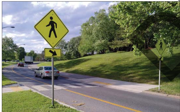
This pedestrian crossing at Broken Land Parkway and Snowden River Parkway has ADA-compliant perpendicular curb ramps.
