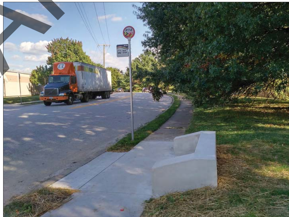
This landing pad and knee wall at an RTA bus stop on Ridge Road in Ellicott City provide an ADA-compliant place for transit users to wait for the bus.
